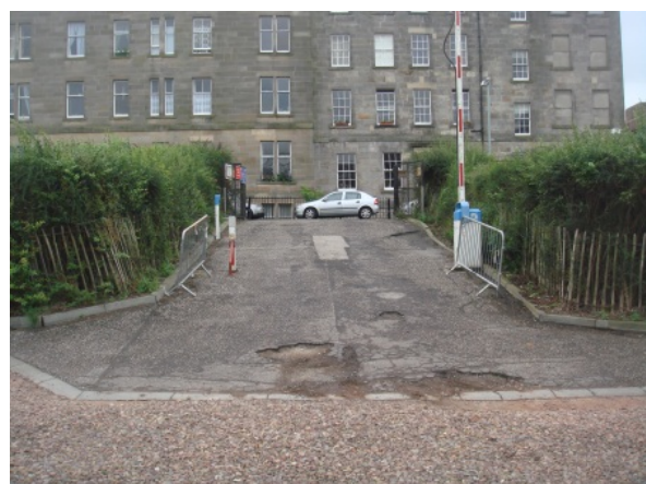
Architecture Building car park entrance
