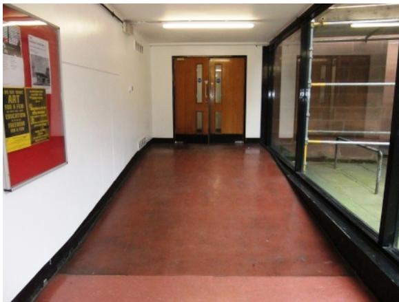
Hunter Building access point
