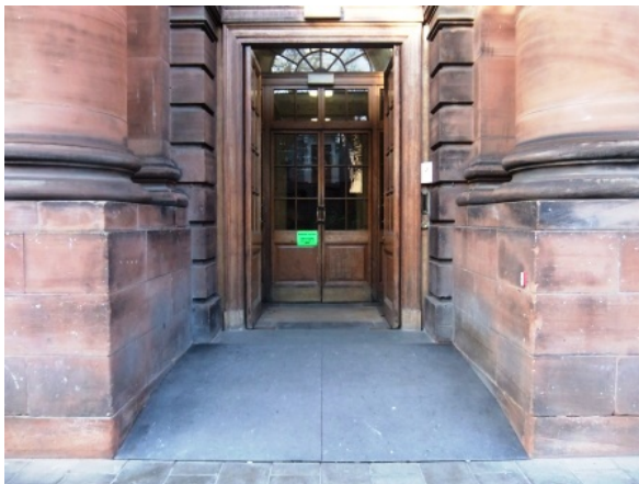
Ramp at Entrance 1
